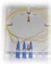
SPLICE BOX WITH PIGTAILS INSIDE
